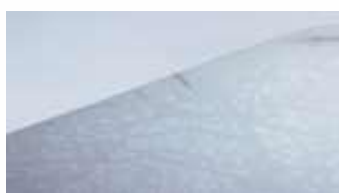
Cracks in Trailing Edge
